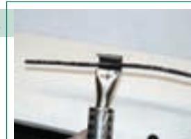
Heat the cable-end with a gas burner or with an industrie-dryer. Remove the worm cable-end.
