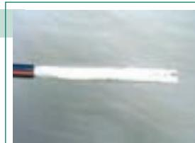
Attach a radial cut, with a cable stripping knife, approx. 15cm from one cable end.
