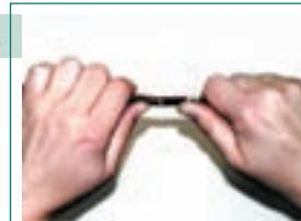
Cut the cable sheath radially approximately 15 cm from one end and the mark of the required length (scratch the corrugated steel tape!) Break the steel tape at those points with care.
