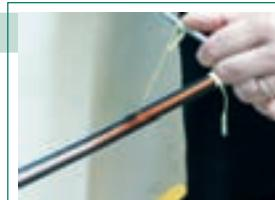
Open the cable sheath by means of the ripcords (vertical to the cable) as long as you need.
